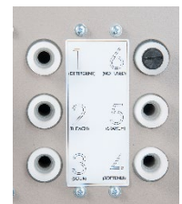
Safe chemical injection
