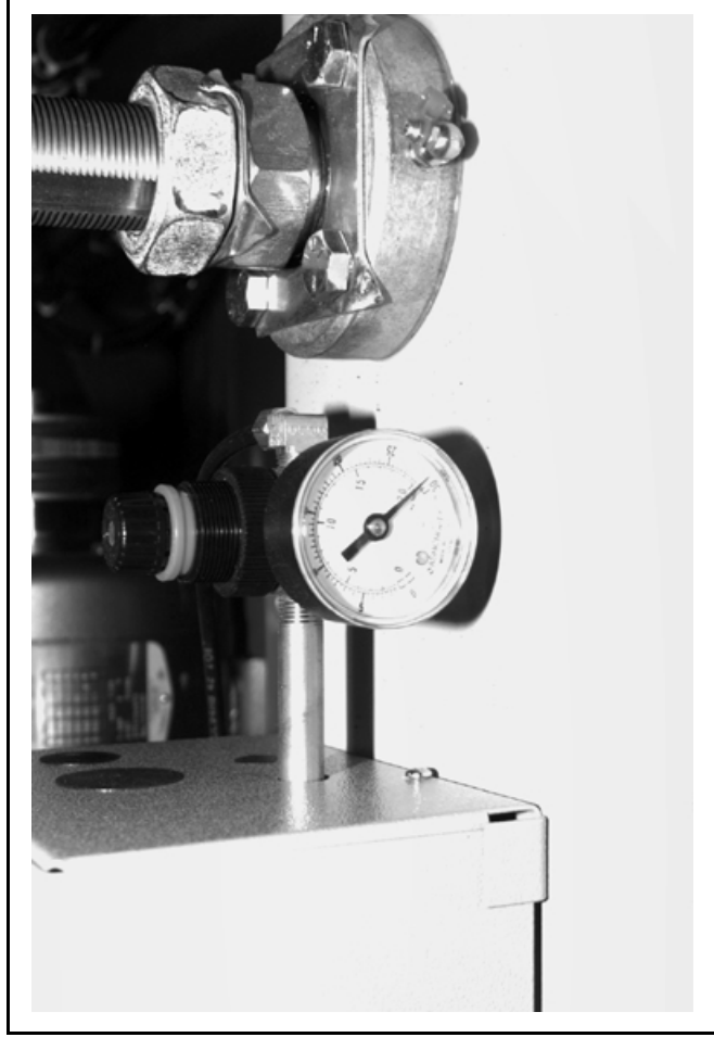
FIGURE 26 (MSSM0201CE) Door Seal Pressure Regulator
