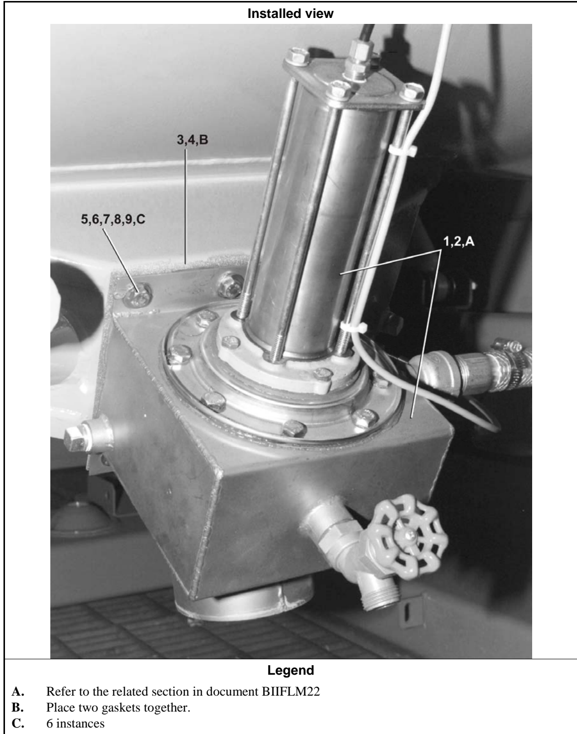
Figure 1: Installation, Drain Valve Body With One Valve
