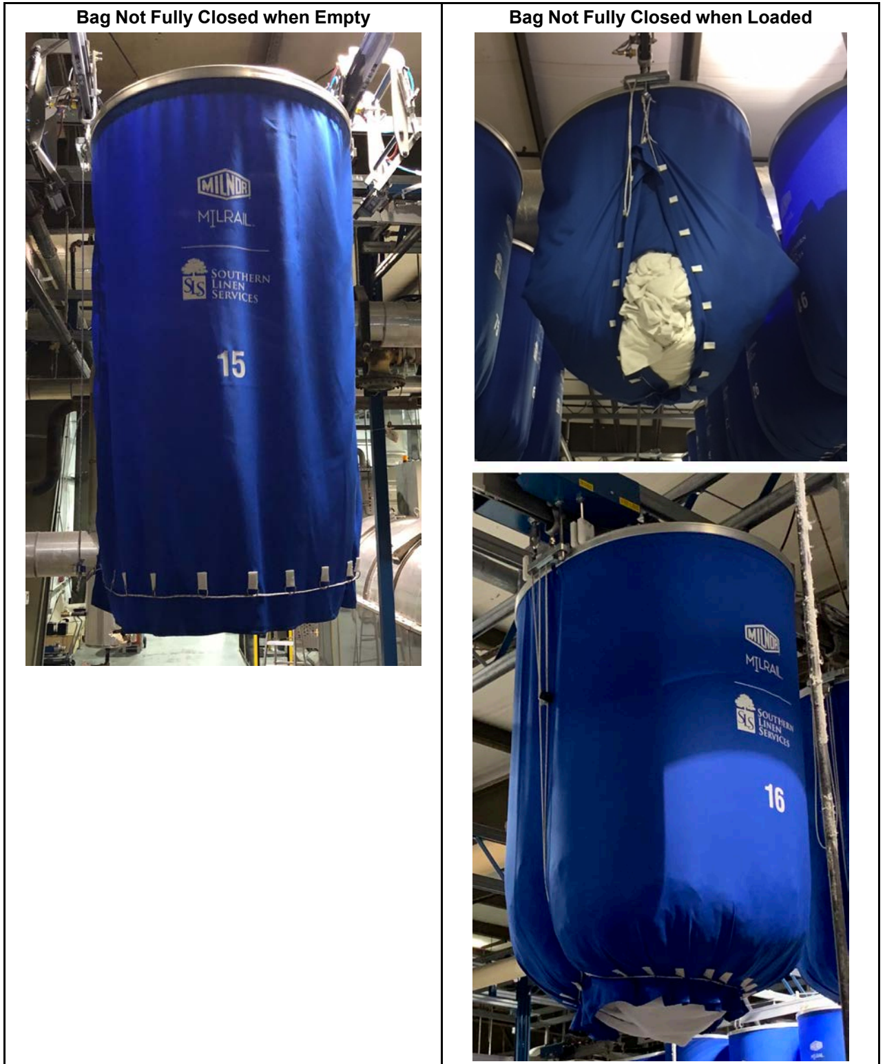
Figure 10. Bag Closing Faults
