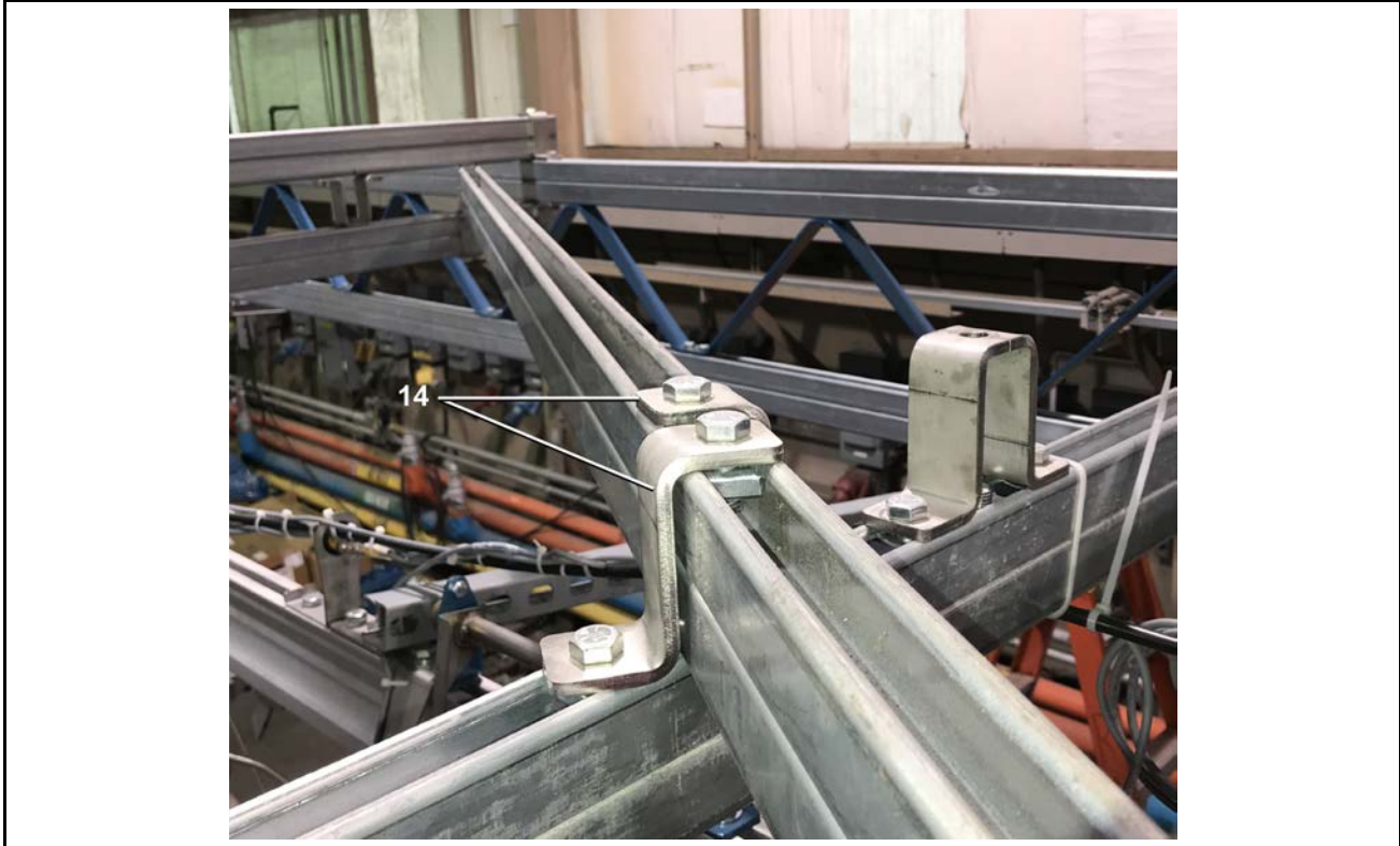
Figure 18. Additional Unistrut Beam Connectors
