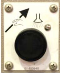
Rakam [Figure] 7: Manuel İkmal Püskürtme Butonu [Manual Supply Flush button]
