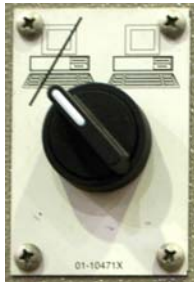
Rakam [Figure] 6: Mildata/Yerel Tercih sviçi [Mildata/Local Selector switch]
