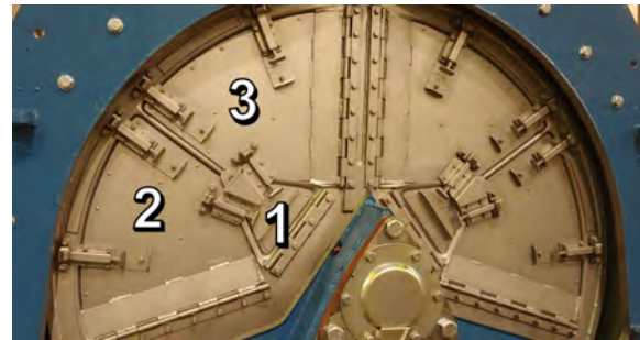
Figure 6. Inner and Outer Doors Aligned for Loading
