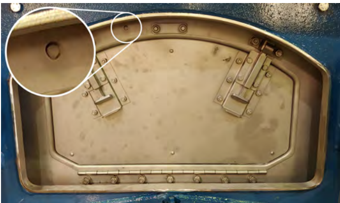
Figure 7. Inner Door Weld Dot
