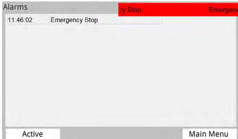
Figure 11. Alarms Menu— Active View
