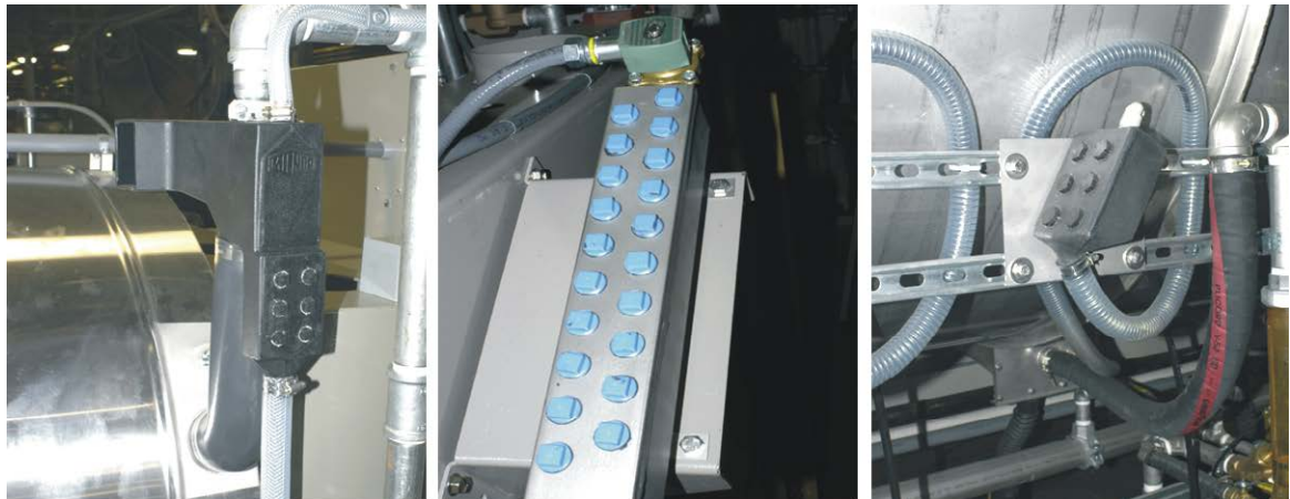
Figure 4: Examples of Manifolds for Chemical Tubes. Your equipment can look different.
