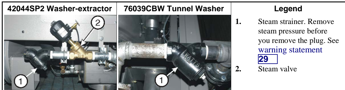
Figure 12: Steam Inlet Strainer. These are examples. Your machine can look different.
