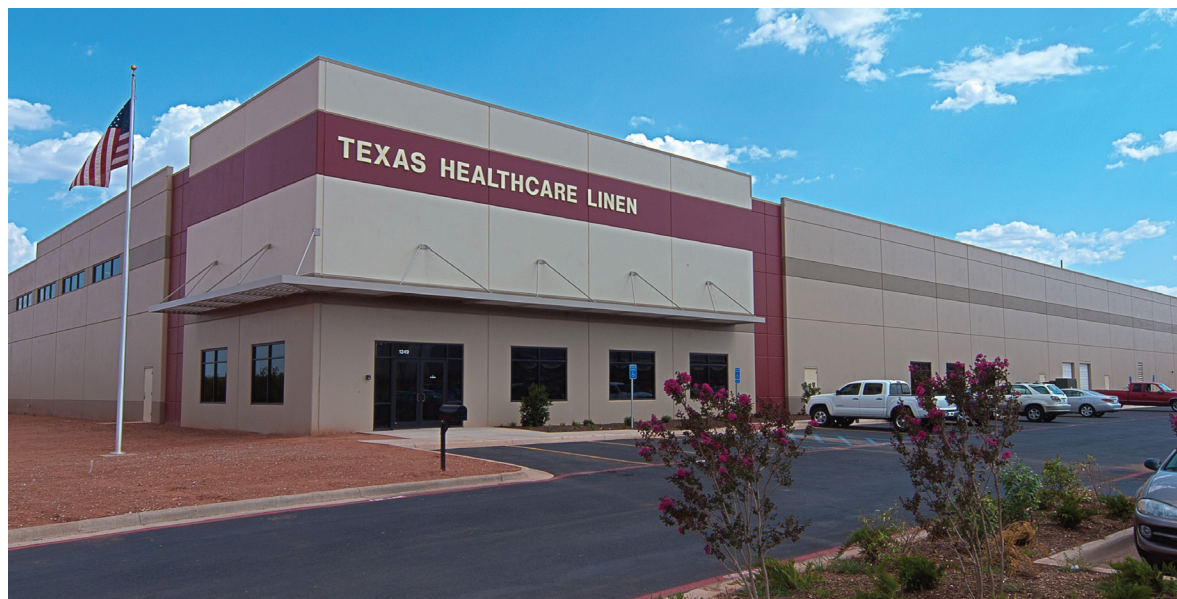
ABOVE: Laundry managers at Texas Healthcare Linen, a hospital-owned central laundry in Abilene, TX, said they wanted a “state-of-the-art facility.” To realize their goal of efficient, high-quality processing, they chose wash equipment from Pellerin Milnor Corp.
