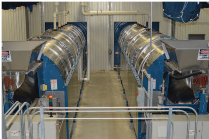
HIGH VOLUMES: Two 10-module PBW tunnels process over 4,536kg/hour
