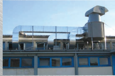
Roof mounted MLF filters are another option.
