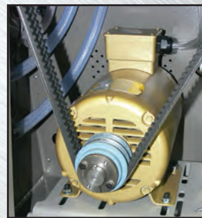
NEMA Premium® efficient inverter-driven motor
