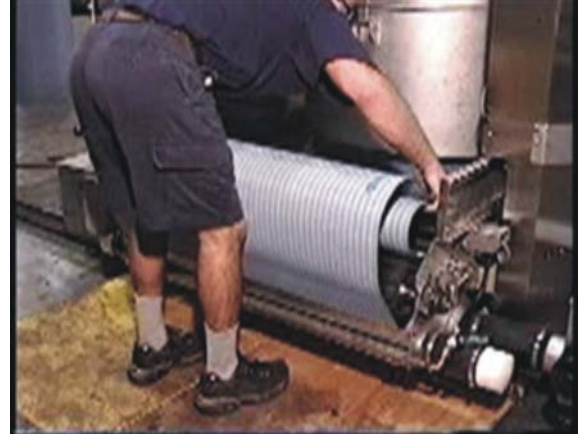
Figure 24: Pulling Belt Through Press from Unload End
