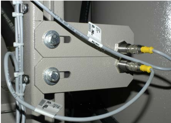
Figure 39: PXSL and PXSB With Brackets Together
